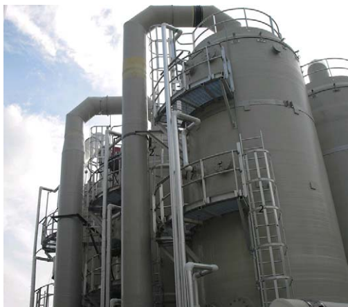
Fig. 2. Bioreactors treating CS 2 -emissions at a viscose plant seeded with extremophile acidophilic microorganisms.
